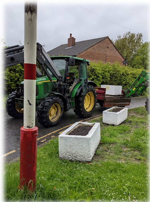
FIGURE 8 – INSTALLING THE COMMUNITY CONTAINERS
