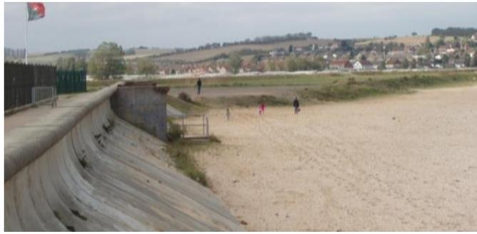
A sea wall on the Sheppey Coast. Coastal defences are the first line of defence against coastal erosion and flooding.
