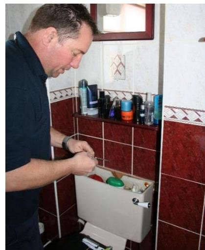
A plumber installing dual flush and a Hippo water saving kit in homes. Saving water in the home means you are less vulnerable to water shortages from drought.
