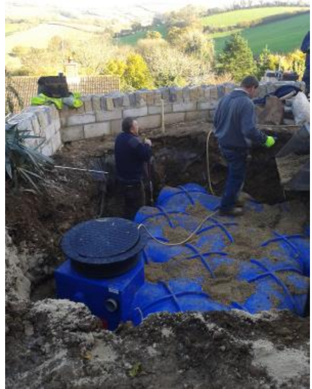
Figure 6 - Installing a rainwater harvesting tank, Ryall, Dorset
